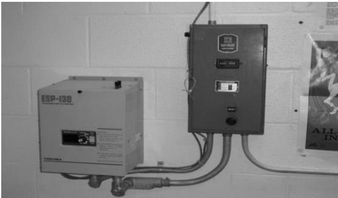
Figure 79: Fan motor speed and power controls
