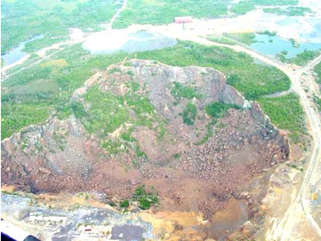
Figure 114: Creighton NHEA system looking east to west. The widths are both approximately 900m. Underneath the surface, trenches go down to a depth of approximately 450m below. (Image courtesy of Vale)
