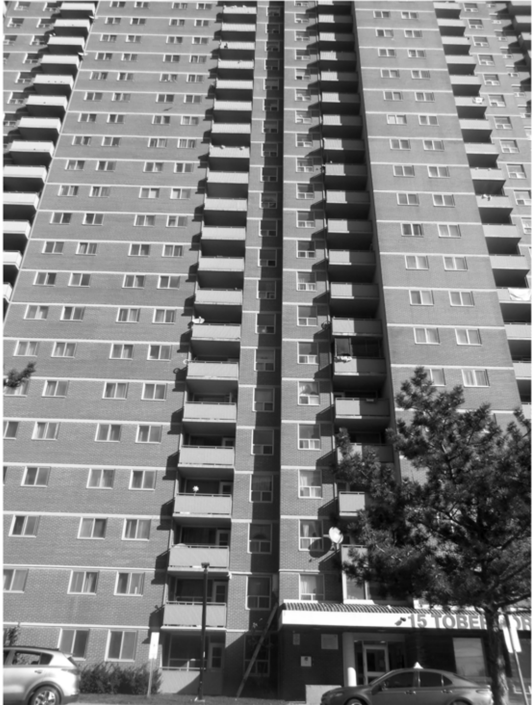
Figure 16 : Tower Facade in Jane and Finch
