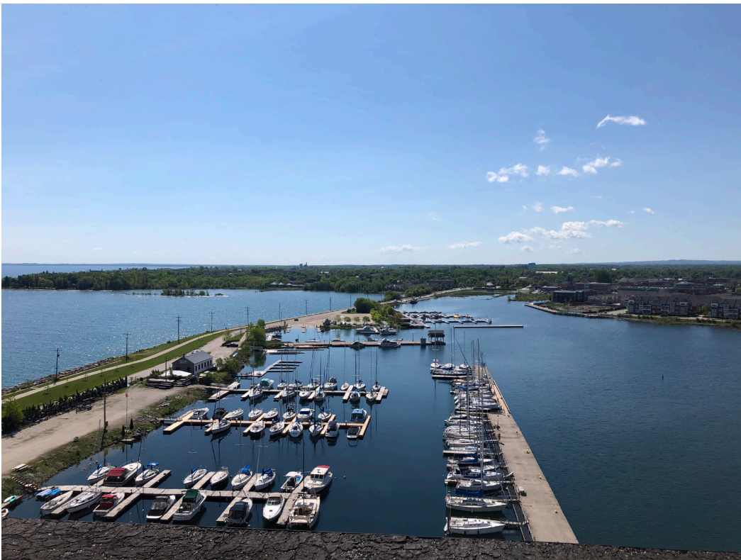
Top 63// South View from Terminals, 2021
