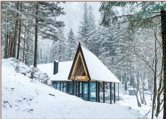
Figure A.0 : Exterior Winter Approach.
