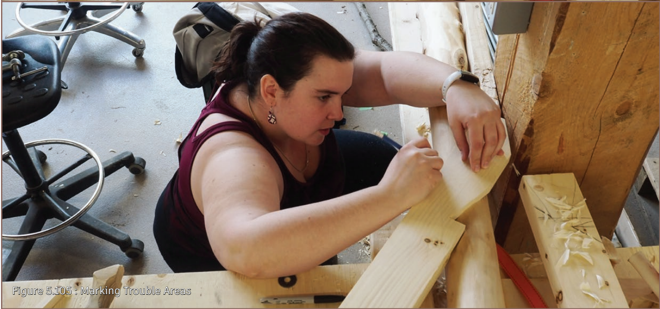
Figure 5.104 : Test Fitting
