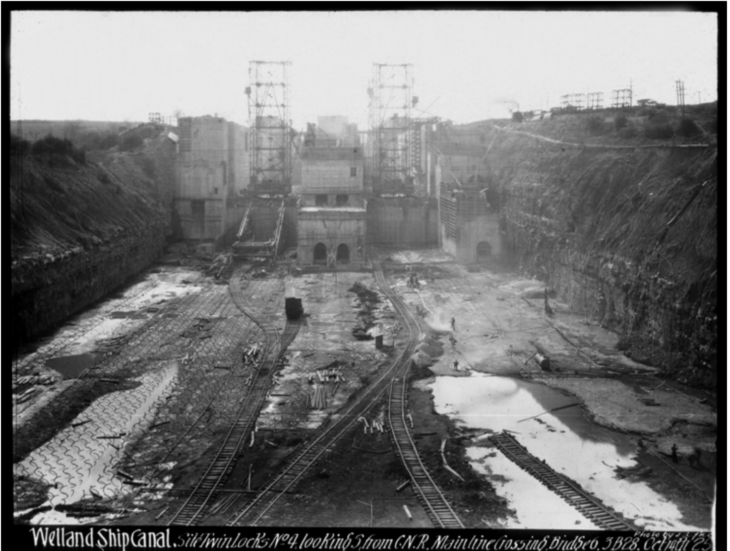
Figure 28: Welland Ship Canal, Site Twin Locks No 4, looking South, from CNR Maintenance crossing Bridge
