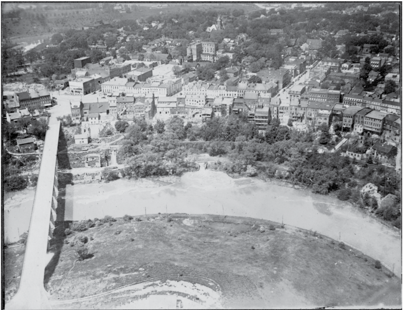
Figure 20: Aerial photo of Downtown St Catharines and with Canal running through
