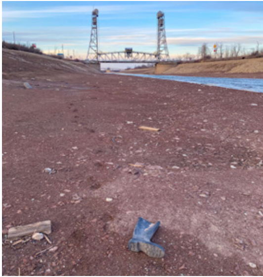
Figure 26: Drained Canal in January, at the base of Lock 4
