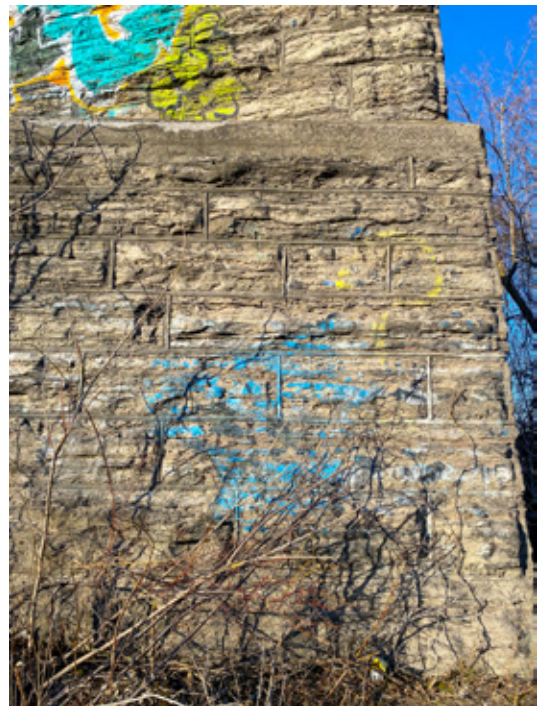
Figure 32: Remnants of masonry construction found along traintracks around Lock 4 Site.
