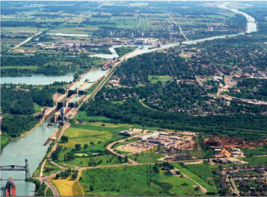
Figure 29: Aerial View of Canal
