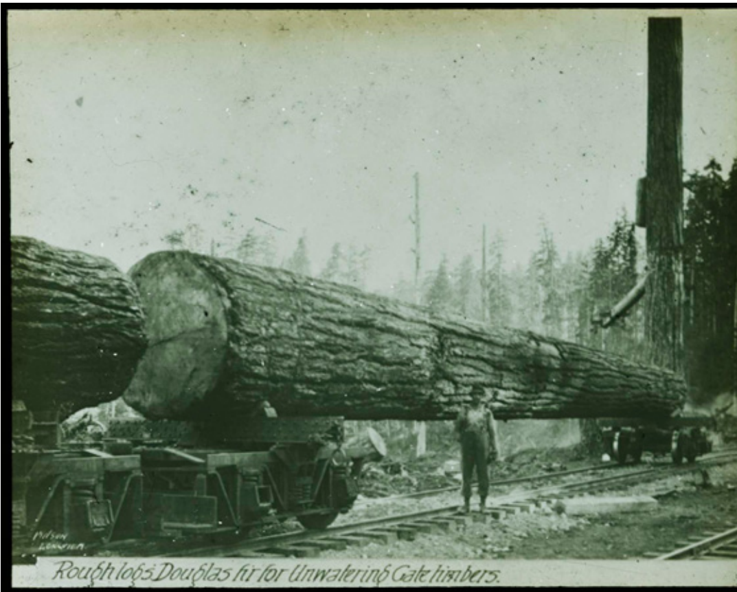
Figure 17: Rough logs – Douglas Fir for unwatering gate timbers, n.d.
