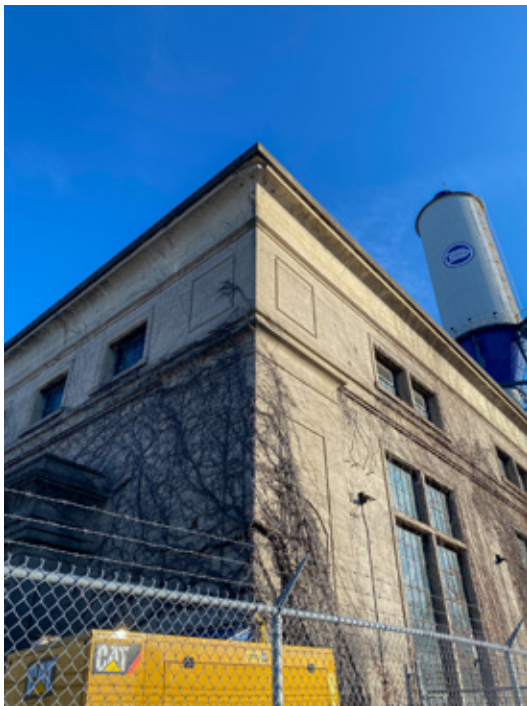
Figure 31: St. Lawrence Seaway Management Corporation Lock 4 Powerhouse building
