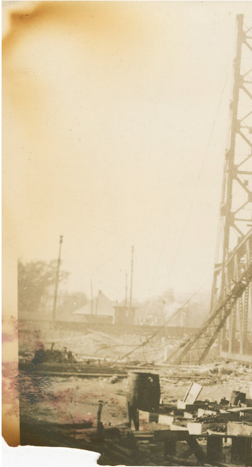
Railway Bridge Construction in Port Colborne Ontario, 1927
