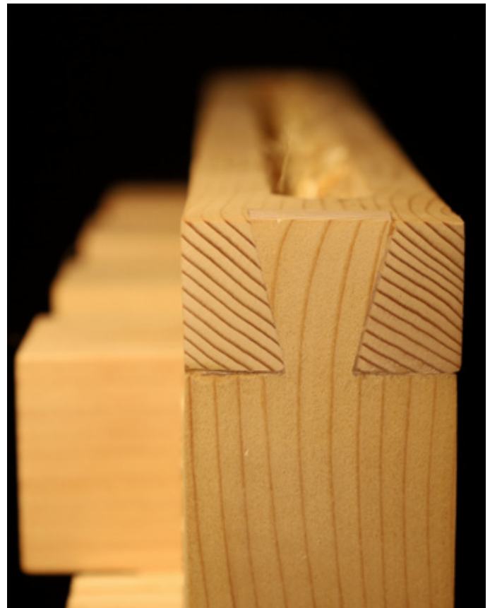
Dovetail joinery holding the case together
