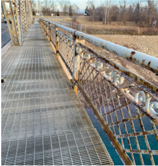
Figure 27: Ornate lattice guardrails along the vertical lift bridge 5
