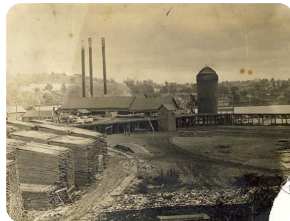
Figures 6-13 IN ORDER FROM LEFT TO RIGHT Historical Photos of notable Parry Sound areas and building typologies
