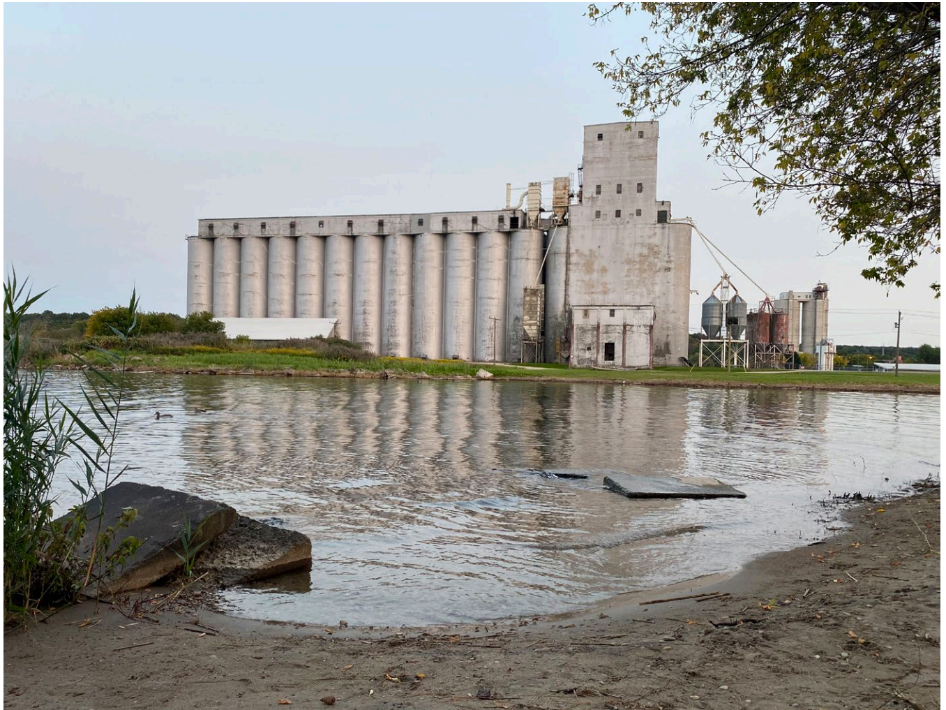
Figure 8: Elevators seen from Kelso Park
