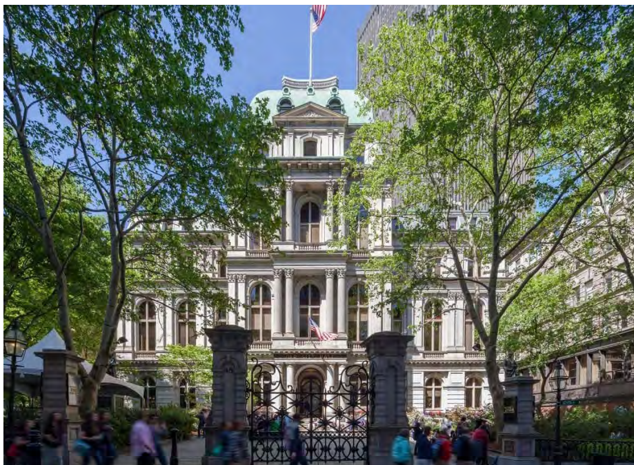
Fig. 52 Old Cit Hall adaptive reuse in Boston, Massachusetts.
