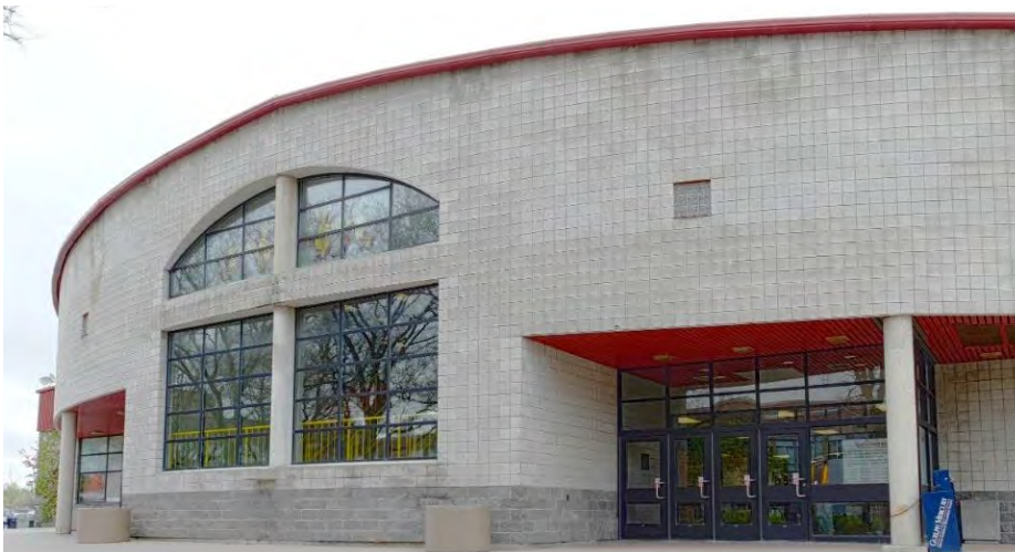
Fig. 22 Gryphon Centre Arena in Guelph.
