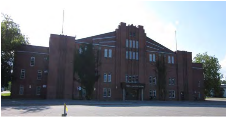
Fig. 60 Verdun Auditorium prior to renovations.
