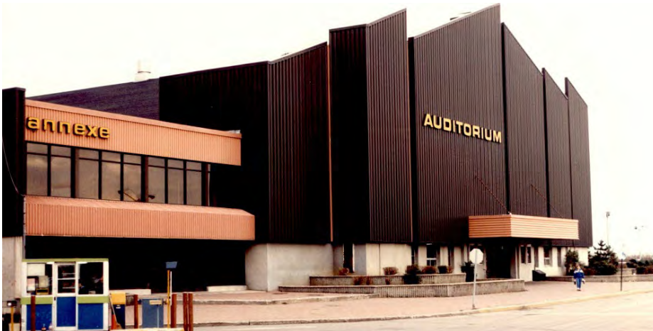
Fig. 61 Verdun Auditorium after first renovation.
