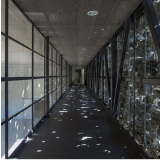
8.16 Dominus Winery by Herzog & de Meuron, showing a speckled lighting effect achieved with a gabion screen. Photographed by Yuequi Li.
