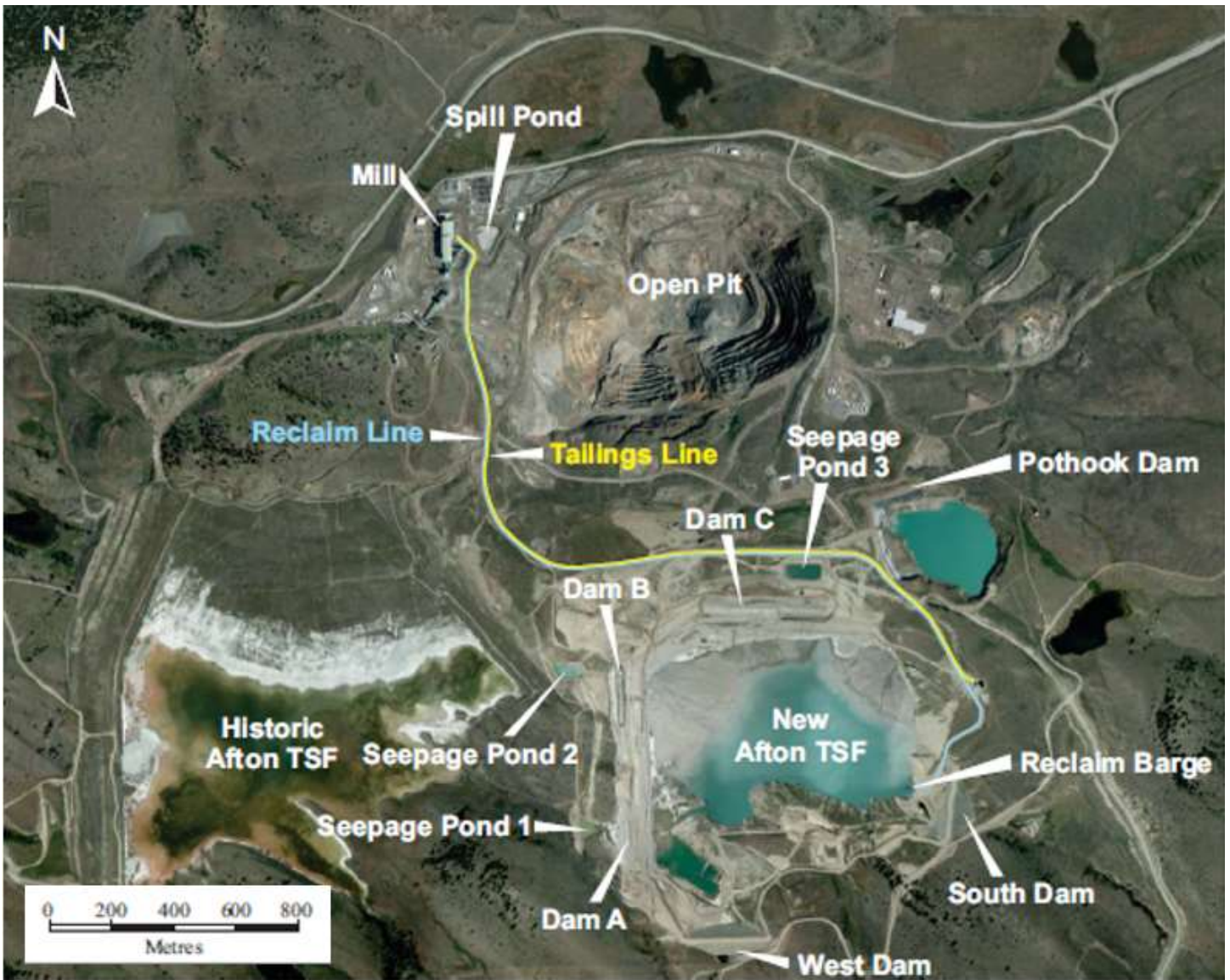
Figure 22. Surface infrastructure of at New Afton Mine (RPA, 2015)
