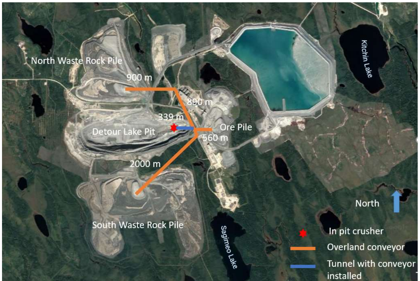
Figure 52. Installation of overland conveyors and in pit conveyors through a tunnel in the pit wall
