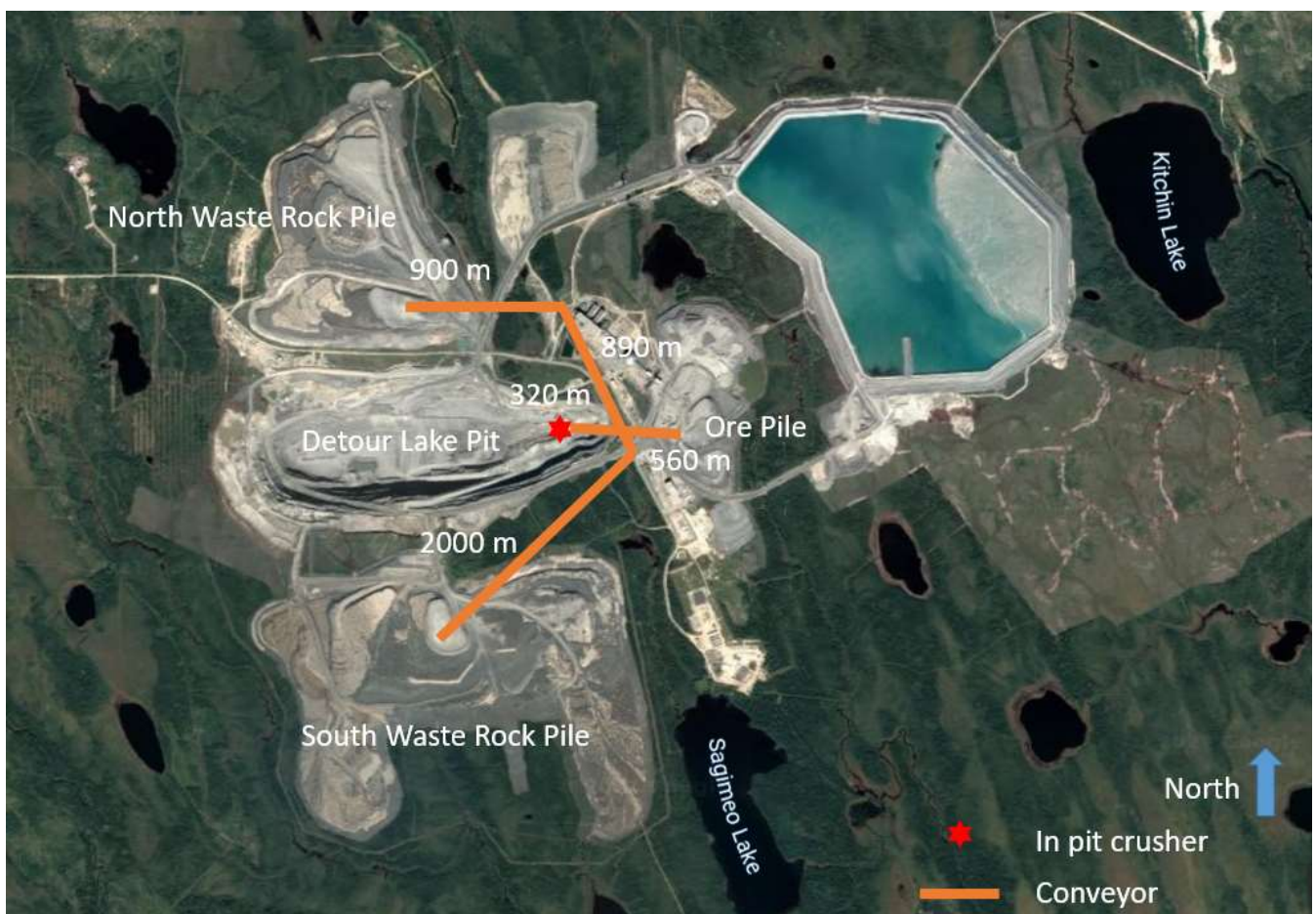
Figure 50. Location of the in pit crusher and path of the traditional conveyors to the various dump points.
