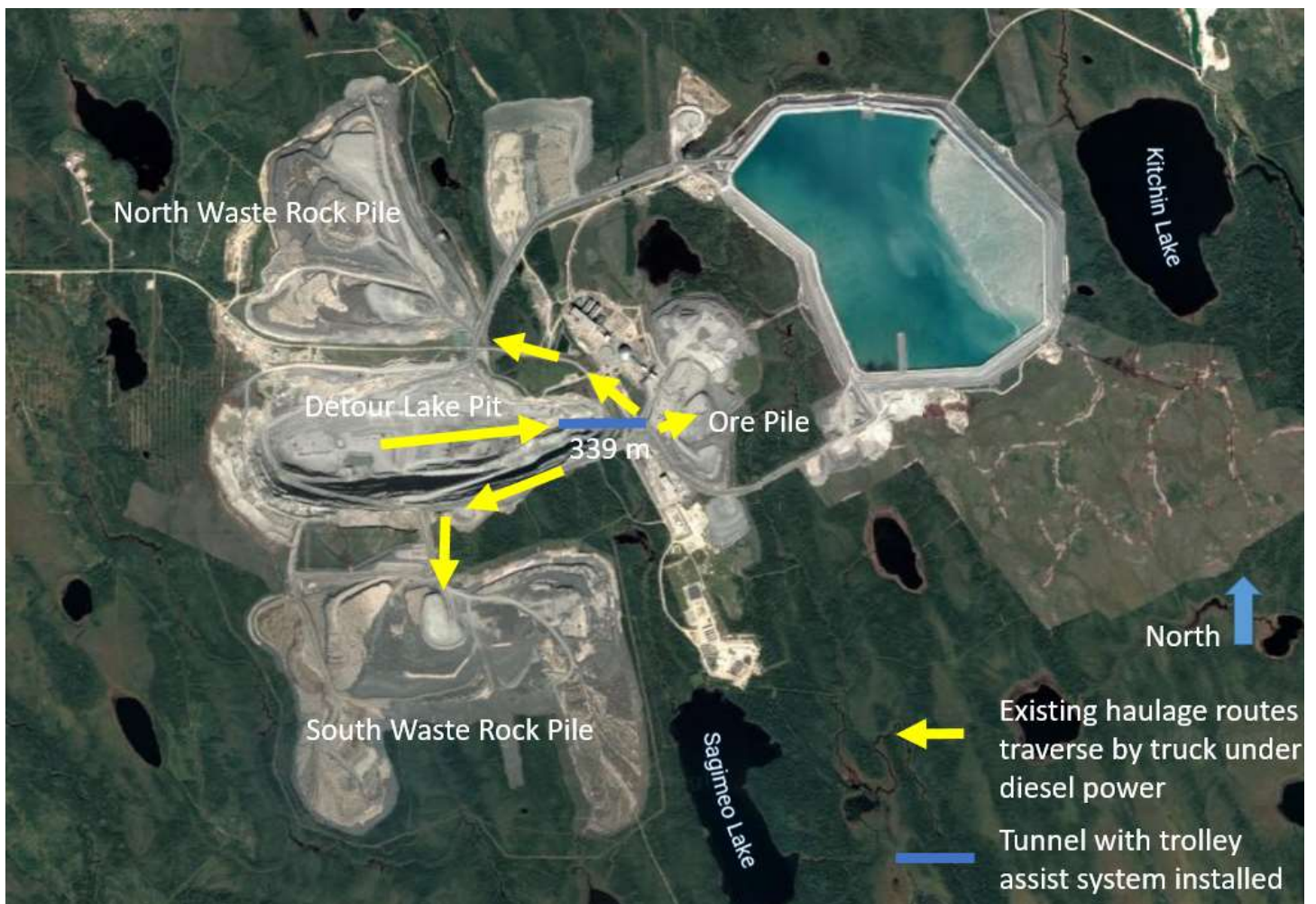
Figure 49. Installation of the trolley assist system through the pit wall via a tunnel in year 2022
