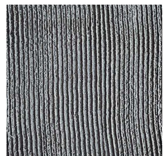
Fig. 79 Combed stucco finish
