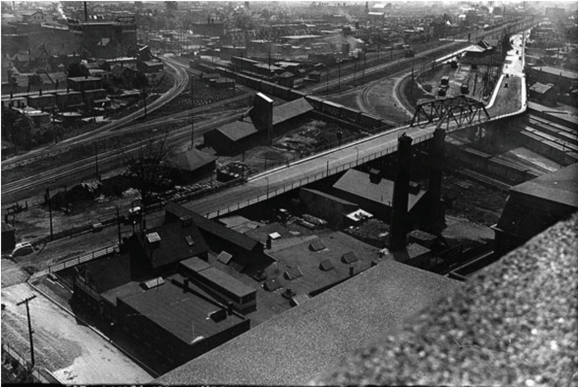
Figure 18: Aerial View of the Railway Intersection.
