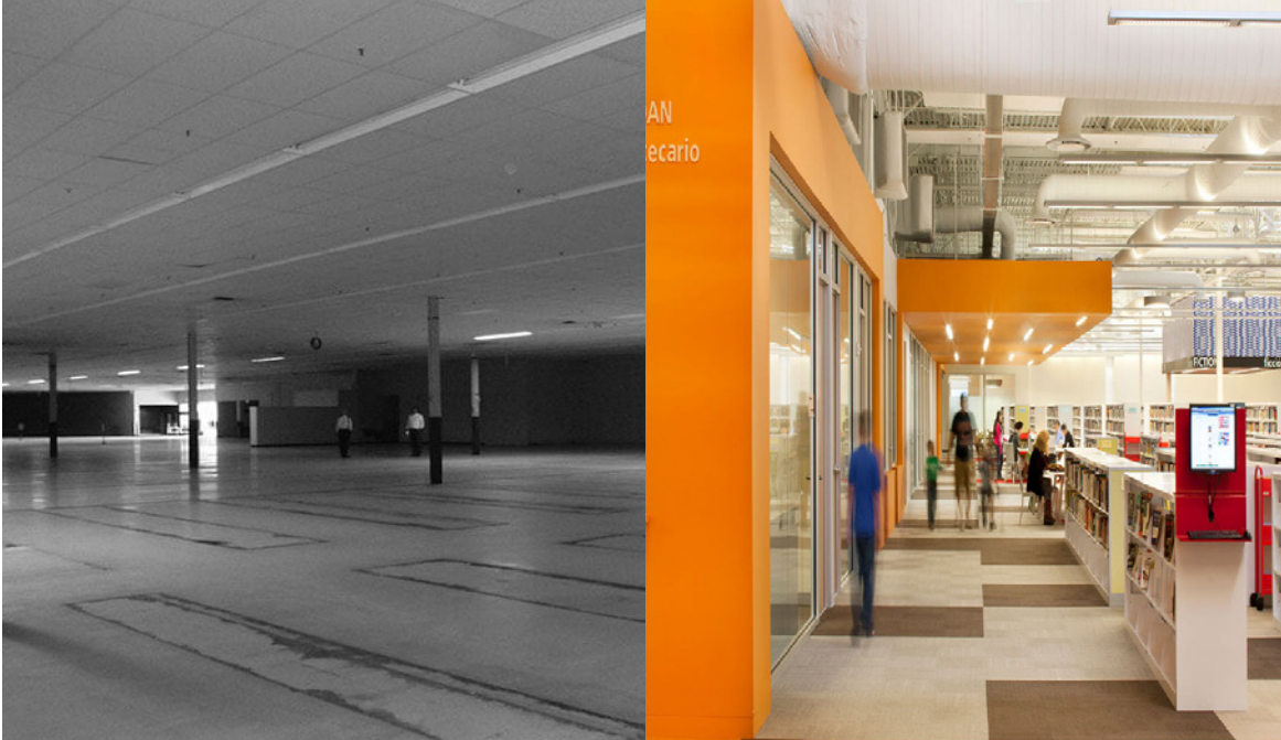
Figure 62 Left: Existing Building Interior Gutted Figure 63 Right: Existing Interior Spaces Painted White.
