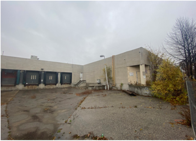
Figure 44: Bay doors of the building.
