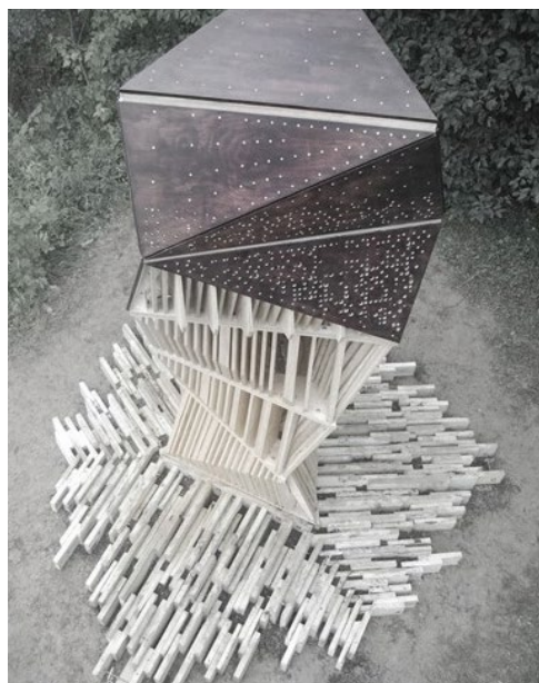
Figure 22 | Bat Tower Interior This photo shows the structures slatted plywood material intended to be inhabited by the bats. [Top]
