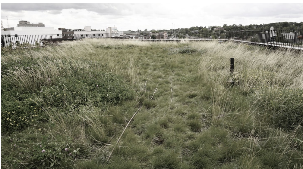
Figure 37 | Laurentian University McEwen School of Architecture Rooftop Garden [1st row]
