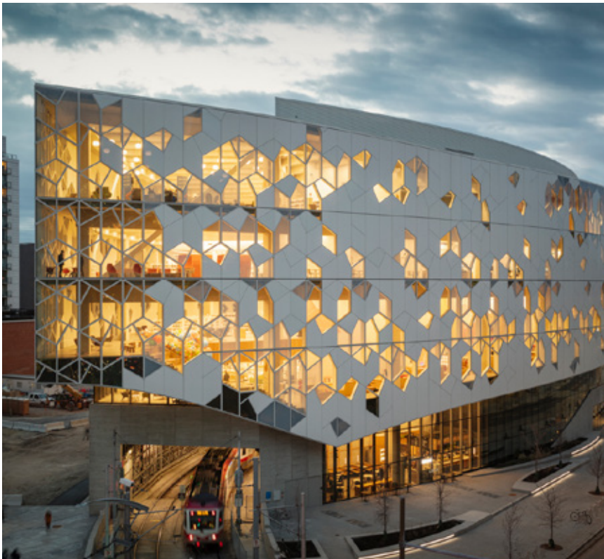
Figure 3.41 Exterior of Calgary Central Library
